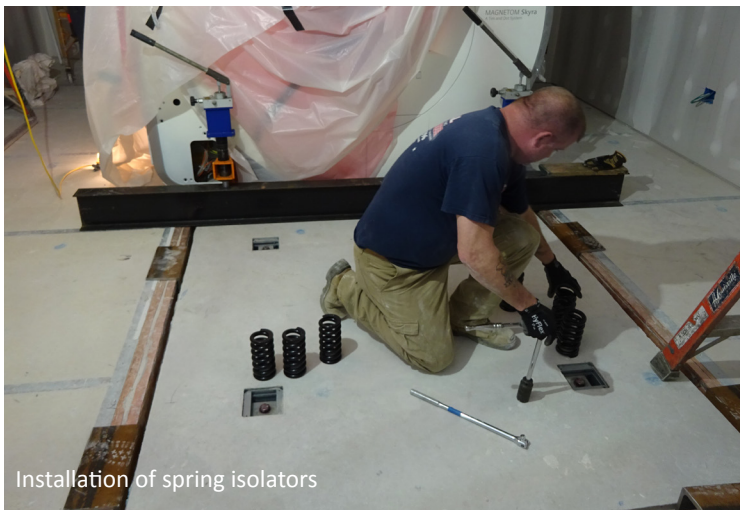
Jacking of floating floor
