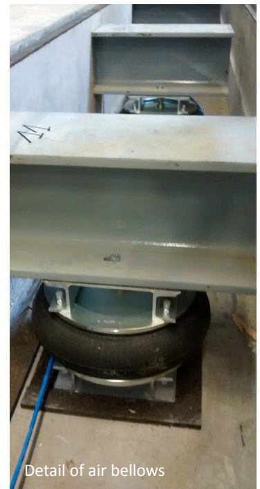
Air bellow installation
