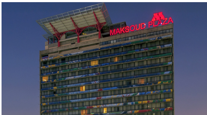
■ [3] Metallic superstructure Maksoud Plaza Hotel, São Paulo [BR] System: CDM-FIX
