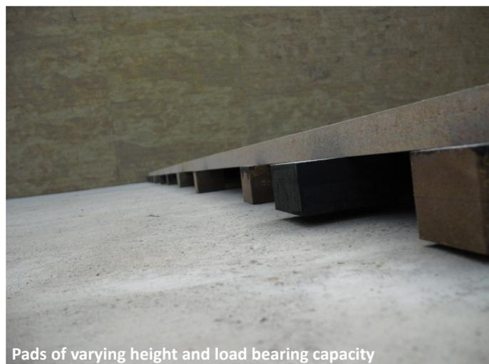
Pads of varying height and load bearing capacity
