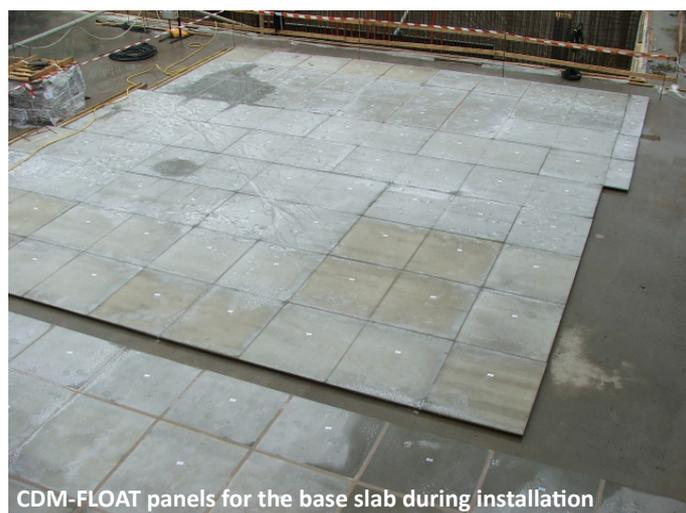
CDM-FLOAT panels for the base slab during installation
