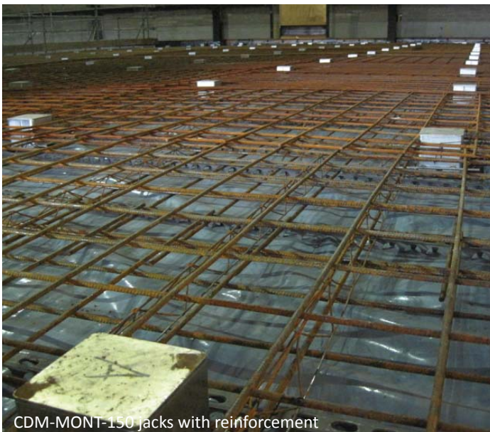
Jacking up a slab
