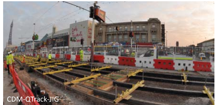
CDM-QTrack-JIG being installed January 2010
