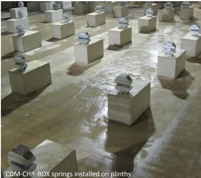
CDM-CHR-BOX springs supporting steelwork in TV Studios
